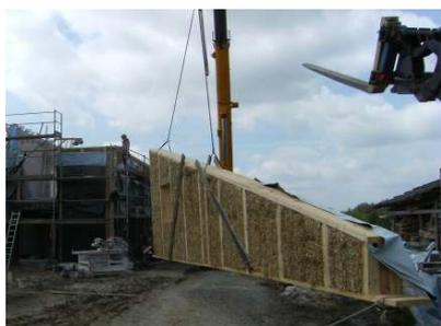
If prefab: Erecting wall elements by crane
