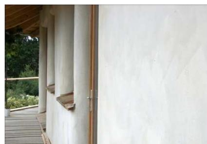
Exterior lime plaster. Rounded soffits. Oak timber piece against moisture at window sill.
