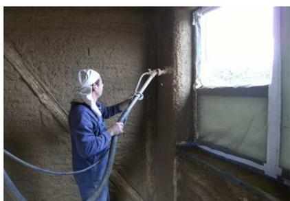
Interior earth plaster with spraying machine. Reed on timber parts. Airtightness with masking tapes.
