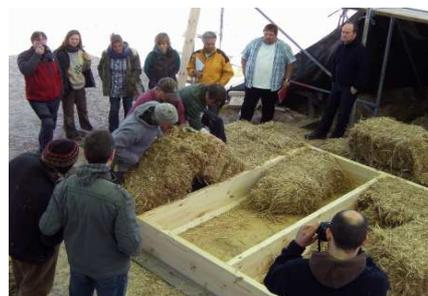
If prefab: After framing, stacking bales, compression done by hand and personal weight
