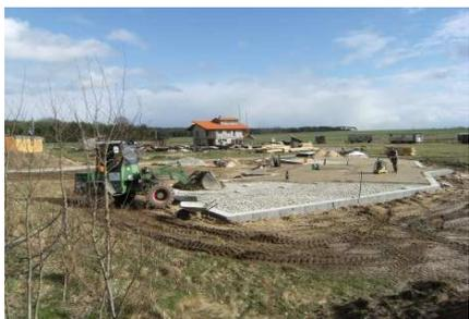
Strip footing, gravel in between, thin layer of concrete as base plate
