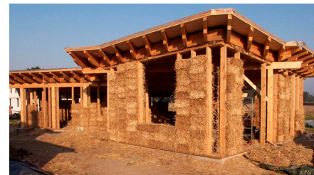
complete straw - walls
