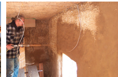
high-pressure plastering
