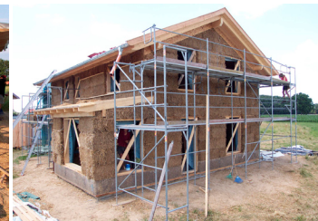
complete straw - walls
