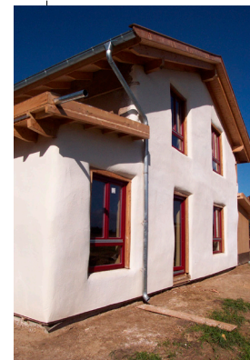
lime-plastered wall
